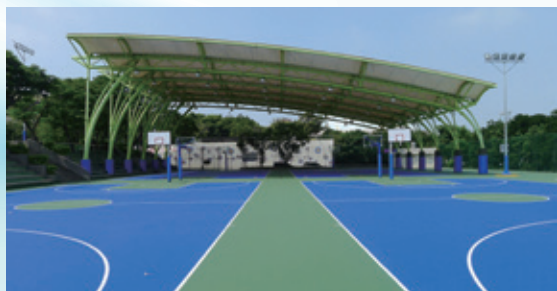
Changhua County Stadium outdoor sports field renovation project- After construction "3-wonder Rice Field Beautiful Path" Bikeway new construction project in Dongshan
