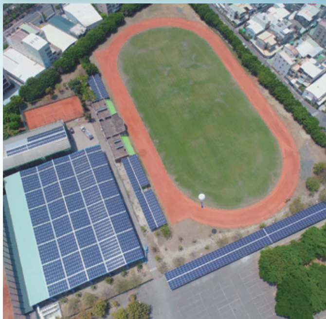
Aerial view of the installation of optoelectronic equipment at Kaohsiung Municipal Sanmin High School
