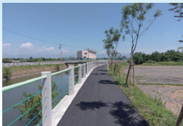
Township, Yilan County- After construction
